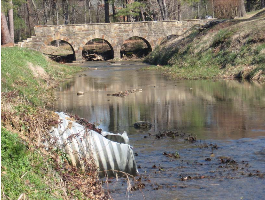
Figure 8 Current photo of NYA Pedestrian Bridge (2008)
